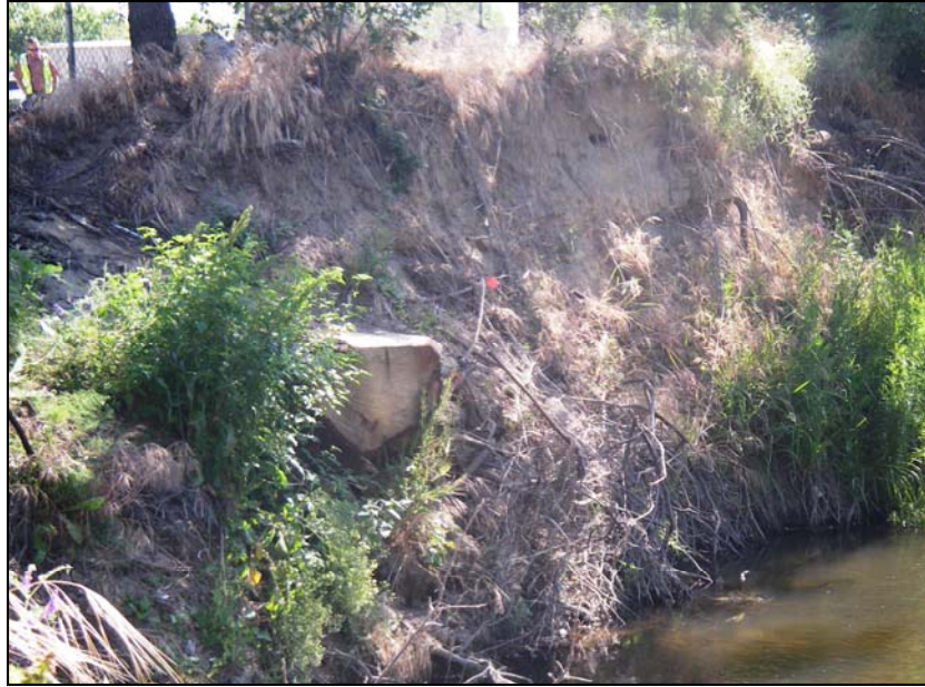
Description: OHWM delineated along Dry Creek in the WWTP, NE aspect.
